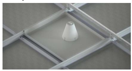
Other services can be integrated with SAS150. Modular lighting can be supported directly from the soffit. Where maximum point loads are exceeded (5lbs) the service must be supported independently or from the grid.
