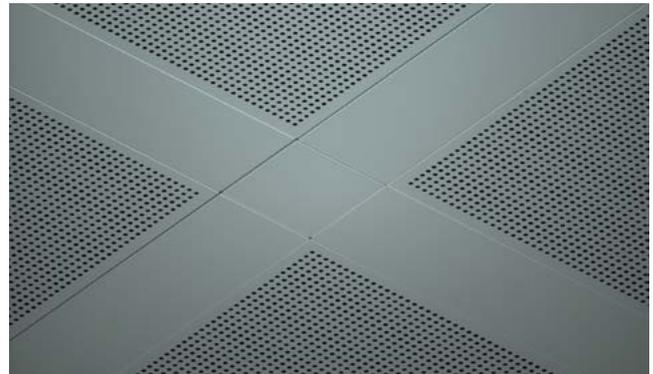
Traditional tartan grid systems make the use of trim strips and crossing boxes suspended from threaded rods and hanger brackets. This detail can be replicated by pressing mock crossing details into the C-Profile. Using C-Profiles instead of crossing boxes provides a far more rigid and durable structure. C-Profiles also provide flexibility to avoid costly bridging around ductwork in the void.
