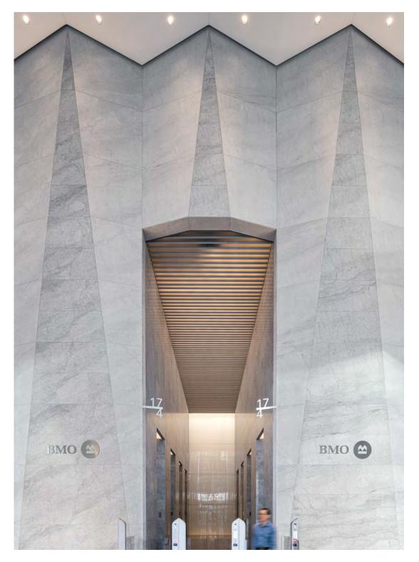
Designed by architects Goettsch Partners, the building's lobby contains feature ceilings above the elevator entrances utilizing SAS's extruded aluminum SAS740 ceiling system. The design required close coordination with the lighting concept to effectively backlight the ceiling membrane. Custom suspension details were developed by SAS to support the profiles at each end, thereby removing gridwork that would have impacted upon the light location and cast shadows.
