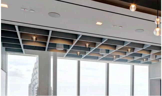
SAS BAFFLE SUSPENSION END BAFFLE CONNECTION PLATE CONNECTION BRACKET FIX THE END BAFFLE CONNECTION PLATE TO SIDE OF THE MAIN RUNNER BAFFLES. SLIDE IN CONNETION BRACKET TO NOGGIN BAFFLE AND LIFT NOGGIN BAFFLE IN PLACE SAS SYSTEM 500 BAFFLE (MAIN ULTRAMICRO S1003 OVERALL RUNNER), ULTRAMICRO S1003 OVERALL PERFORATION Ø0.039" [Ø1.0mm] TO PERFORATION Ø0.039" [Ø1.0mm] TO ACHIEVE 03% OPEN AREA, FINISHED ACHIEVE 03% OPEN AREA, FINISHED PPC RAL 7024 30% C/W ACOUSTIC PAD PPC RAL 7024 30% C/W ACOUSTIC PAD
