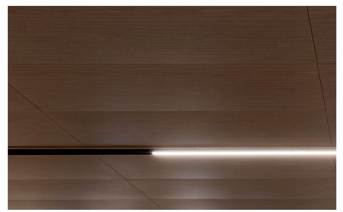
The fully downward accessible torsion spring panels with a concealed grid allows for easy access to the building mechanicals without losing the architectural aesthetics. Additionally, continuous micro perforations provide Class A acoustic absorption, providing a wood-grain appearance with superior acoustic performance as compared to solid wood.
