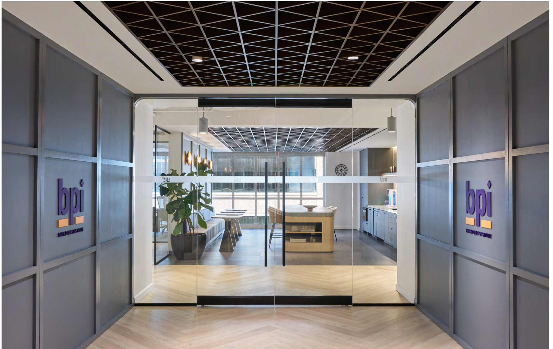
The design called for a ceiling system to visually transition from one area to another, completed by a gypsum perimeter margin.
