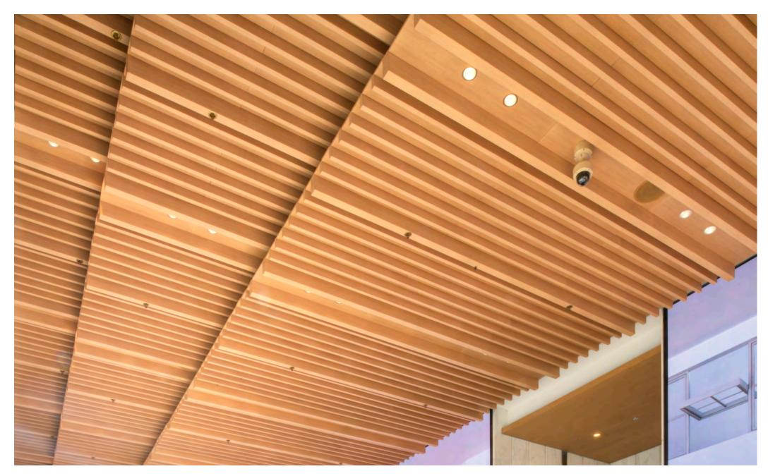
To deliver the geometric ceiling design SAS utilized formed and extruded baffle sections in two sizes, which were supported from our Emac primary grid system. The ceiling membrane then completed with infill panels supported directly via the baffles on each side, thereby removing the requirement for a sequential installation process.
