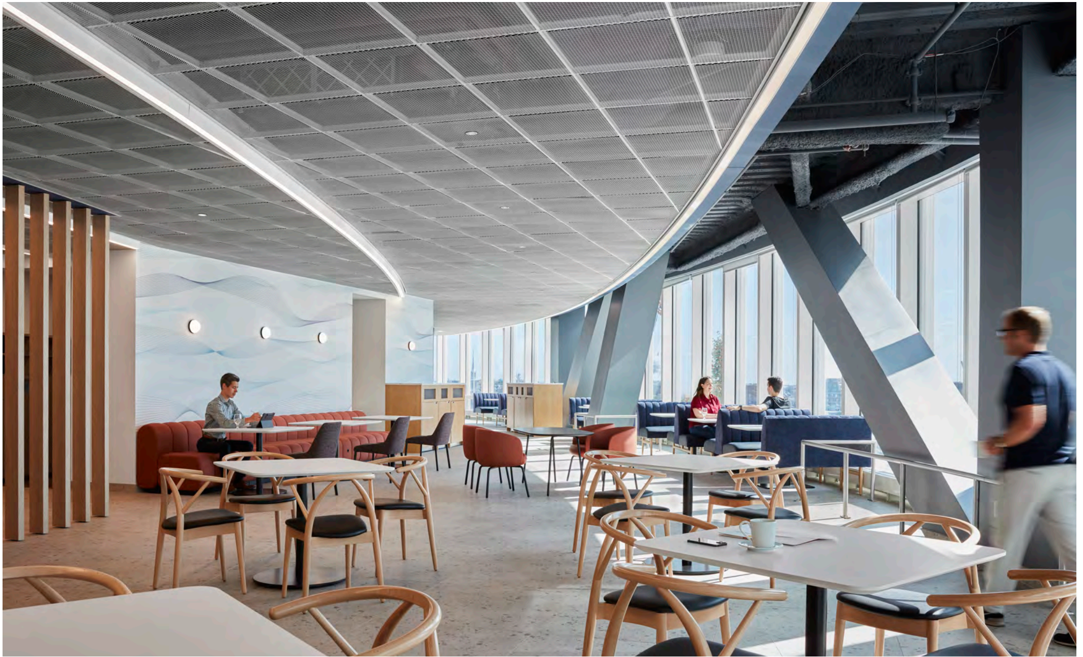
SAS International worked closely with State Street Corporation's fit out architect, Corgan, to specify the SAS130 expanded metal mesh ceiling system in both a white and violet blue color, installed on a fully finished, color matched 9/16" tee grid.
